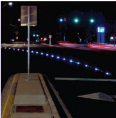
Figure 2: LED Raised Pavement Marker installed at intersection to guide turning movements.
